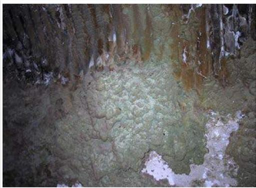
**Figure 3.** Heavy ash deposition (slagging) on radiant furnace walls.
